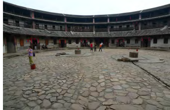
Figure 18: Fujian Tulou, interior. © Lee Ho Yin.
